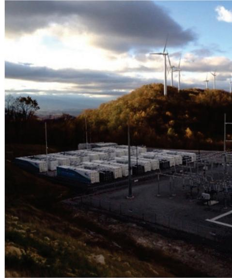
*32MW storage system at AES Laurel Mountain wind generation facility is the largest lithium ion battery project of its kind in commercial operation*
