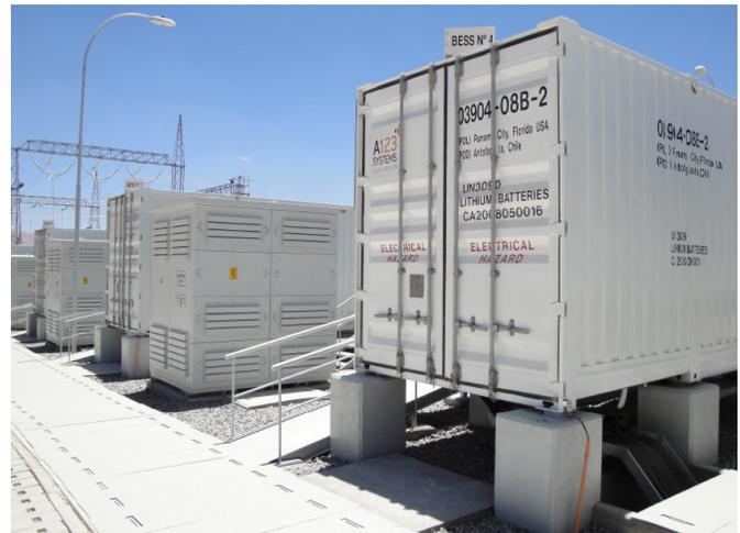
Fig. 1, photo of multiple SGSS units operating in a 12 MW grid storage system
